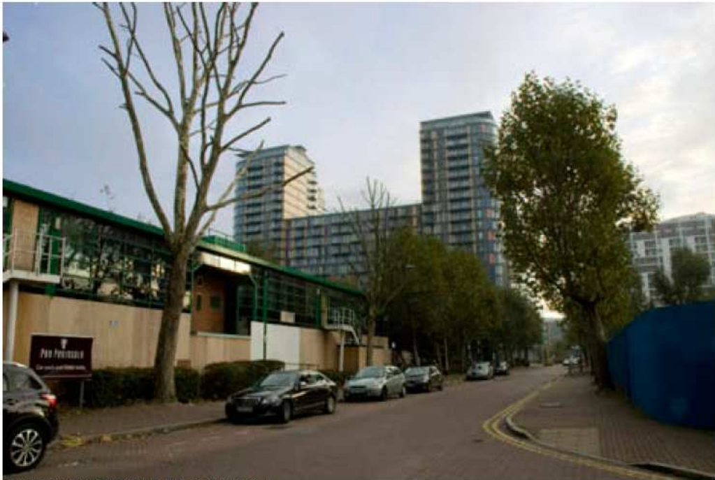
Existing View from North-West of Building
